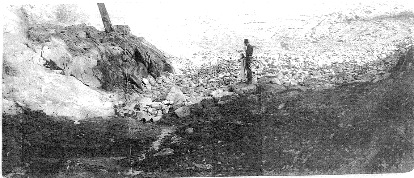
Toe area after placement of the riprap protection.
