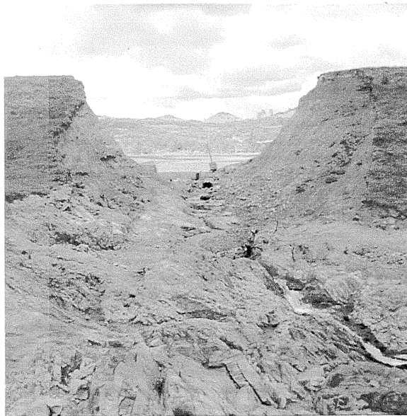
Breach showing extent of sloughing on the sides.
